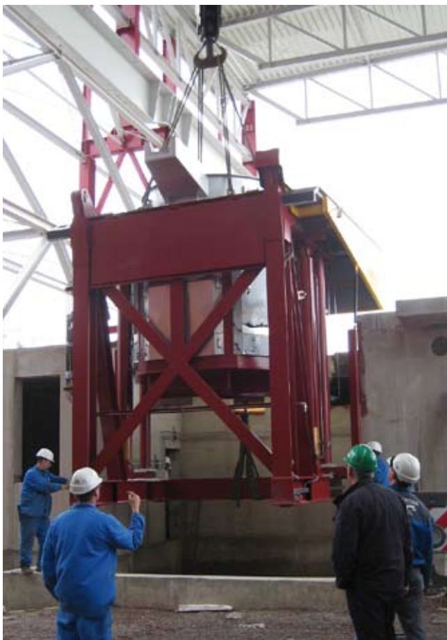
Maximum precision is required during the installation of a furnace
