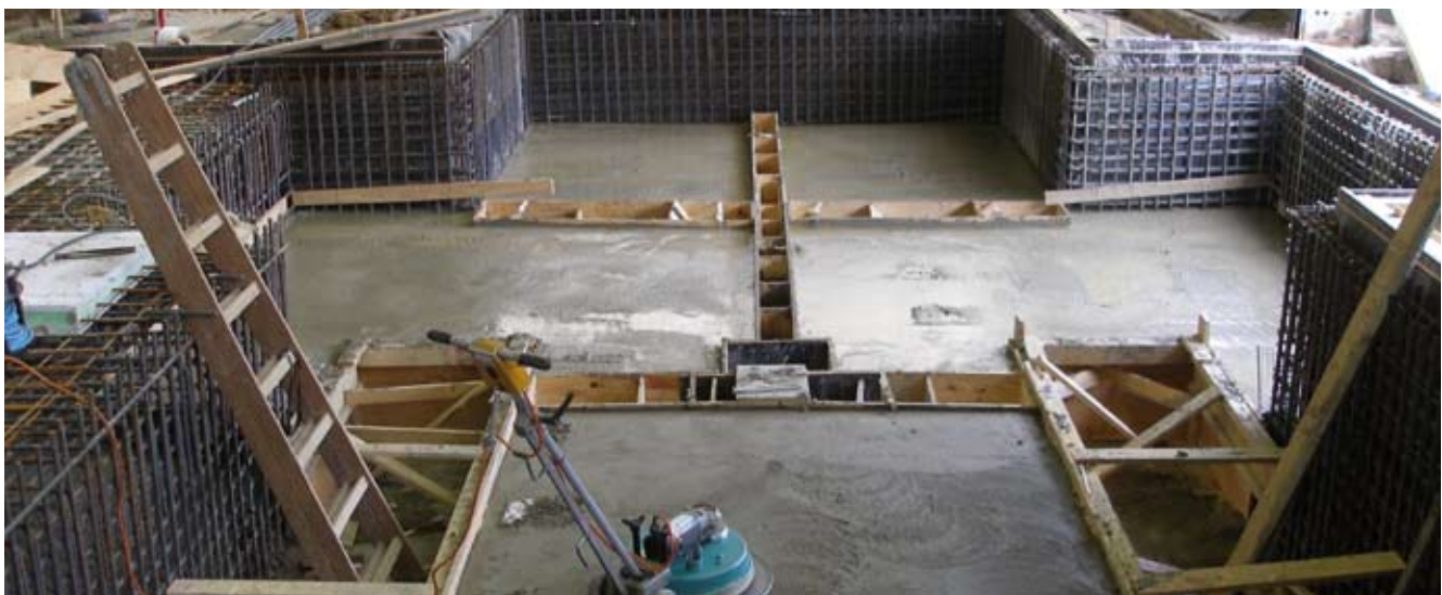
Foundation work for the new machining centre
